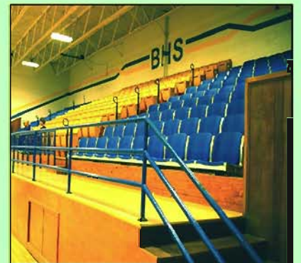
New stadium seating gives the gym a cost efficient facelift.
