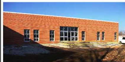
McKinley School addition, new entrance
